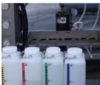
Initial and final Cleaning system
